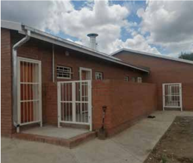
A completed Nutrition Centre at Tharollo Primary School in Fezile Dabi, Free State.
