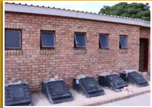
AASA ablution structure in Blouberg, Limpopo
