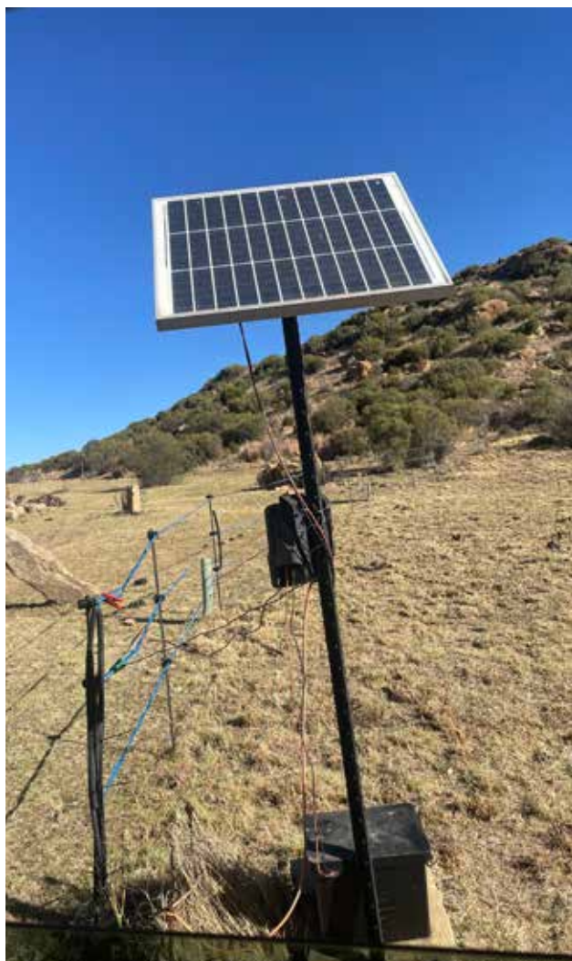
Solar-powered electric fence.
