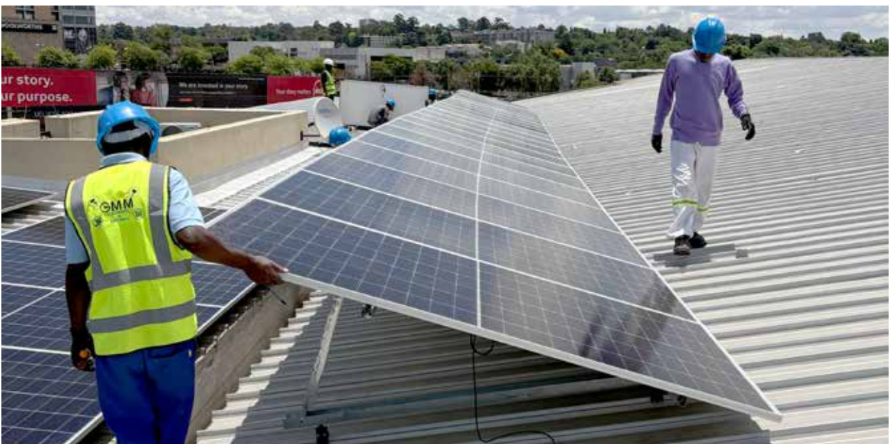
KT Office Solar Panel installation.
